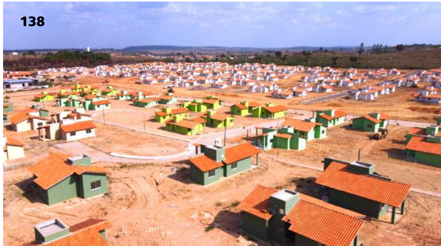
Fig. 138: A drone photo of the construction work completed by 2023.
