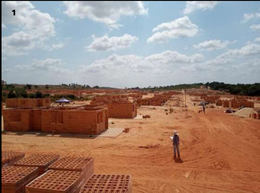
Fig. 1: Construction site of the resettlement of Piquiá de Baixo, the future Piquiá da Conquista, in September 2020.
