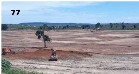
Figs. 75–83: The clearing of the land (drone photograph); construction site sign; sheep foot roller; earthworks and land cuts; rain arriving at the site; excavation of a weir to retain sand and water during rain; surveyors and the advisory team; leveling of the terrain by a patrol; a view of the earthwork hill and heaps of slag for temporary pavement of the streets, 2019.
