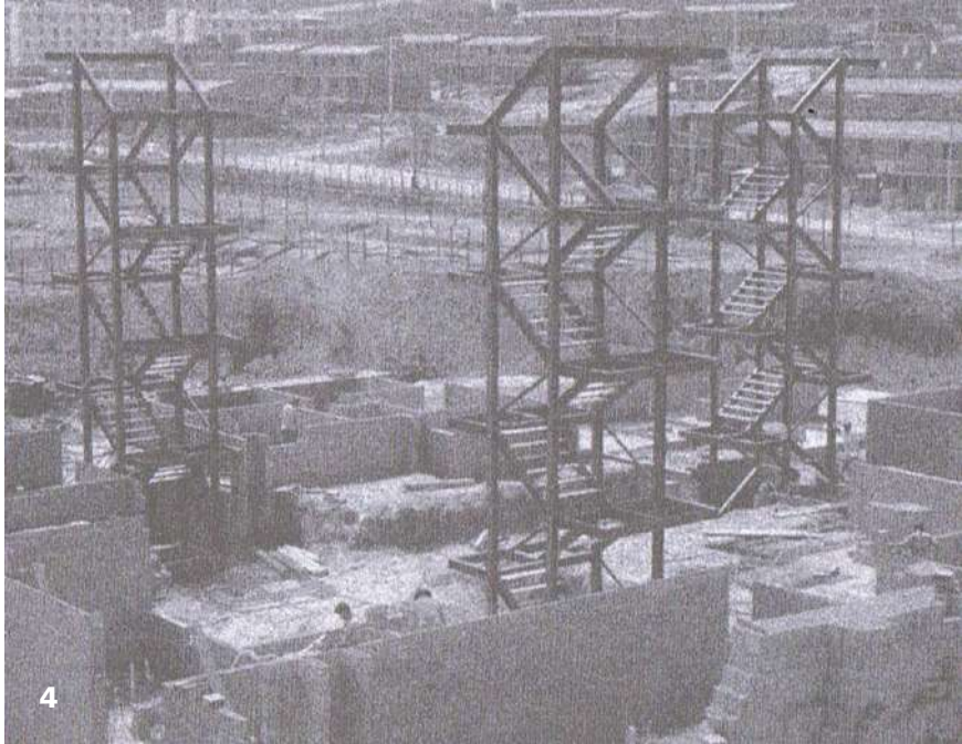
Fig. 4: Construction of the União da Juta Residential Complex, showing the prefabricated steel stairs already set up at the onset of the work. USINA CTAH, União da Juta Construction Association, affiliated with the Landless Workers Movement for East São Paulo 1 (Movimento Sem Terra Leste 1), linked to the Union for Housing Movement (União dos Movimentos de Moradia). São Mateus, SP, 1992-1998.
