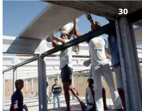
Fig. 30: Manual assembly of a FAEC school in Salvador, 1987. Unspecified location.
