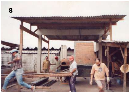
Figs. 5-12: Self-organised collective building projects executed with technical assistance using moulds of 'argamassa armada' in the Vila Nova Cachoeirinha neighbourhood, outskirts of São Paulo, 1992. The 'argamassa armada' elements were produced in a partially industrialized process, in a plant set up with rudimentary equipment on the building site.
