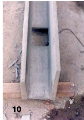
Figs. 5-12: Self-organised collective building projects executed with technical assistance using moulds of 'argamassa armada' in the Vila Nova Cachoeirinha neighbourhood, outskirts of São Paulo, 1992. The 'argamassa armada' elements were produced in a partially industrialized process, in a plant set up with rudimentary equipment on the building site.
